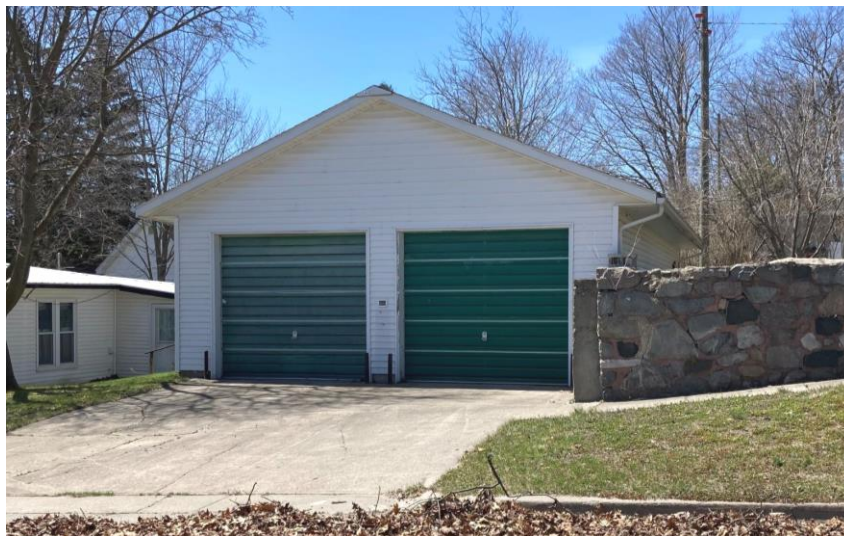
Photo of 401 Antrim St. garage taken on 5-4-2022
