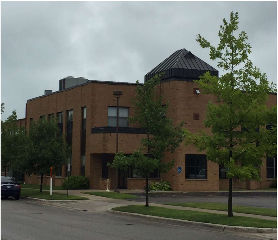
PF – Public Facilities, Charlevoix County
