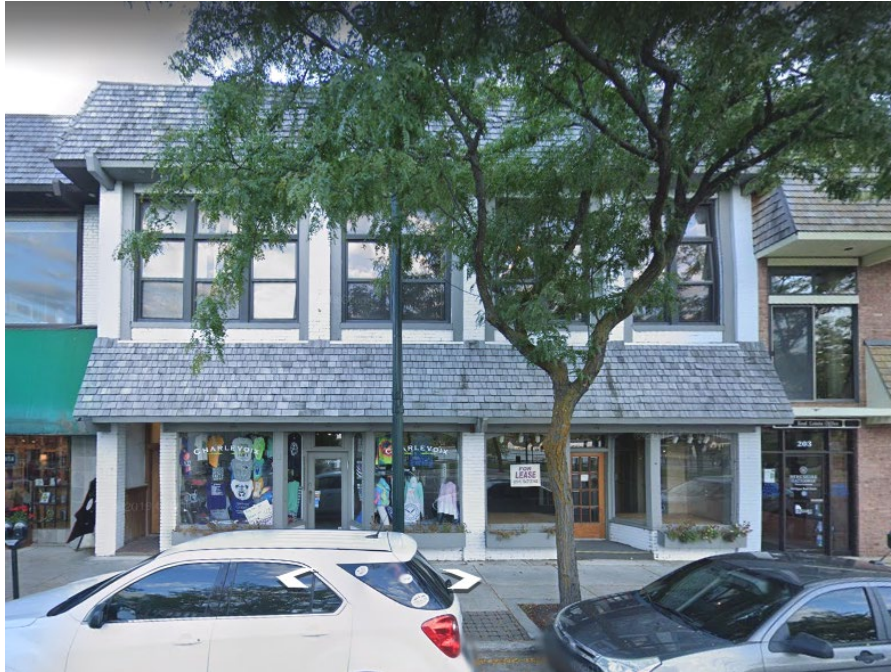
205 Bridge Street Google Earth photo captured on 9-6-2022
