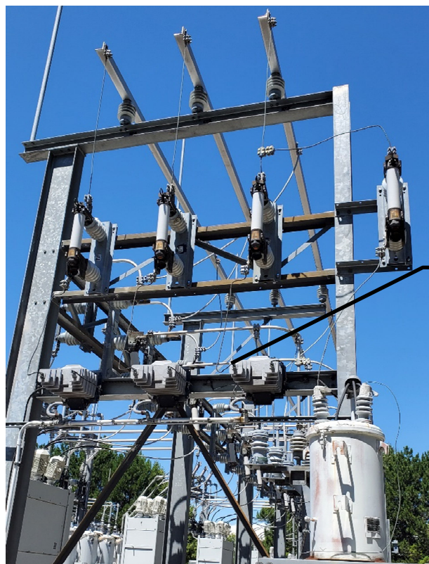
Bus #2 PT's – Bare Copper Jumpers No Wildlife Protection
