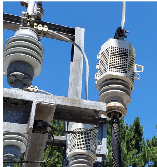
Circuit Riser – Unjacketed Cable, Porcelain Terminations Undersized Neutral to Substation Ground
