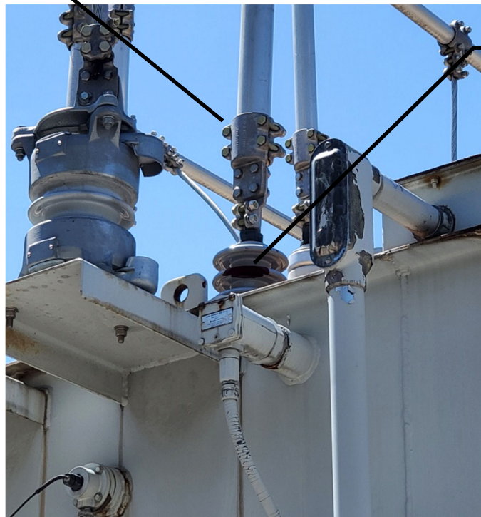
Transformer #1 – Cracked 15kV Bushing
