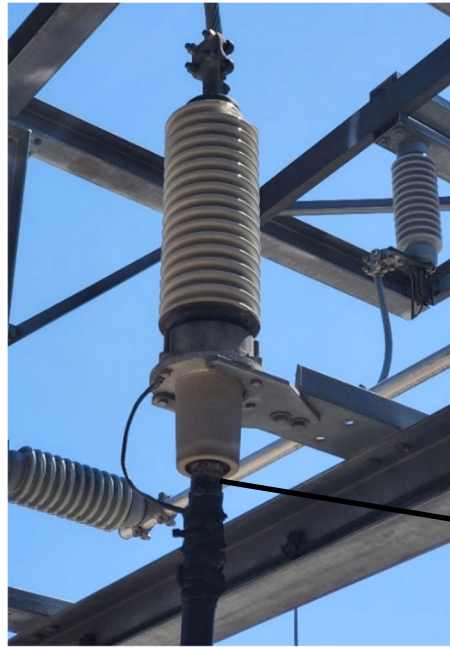
46kV Cable Termination
