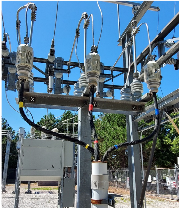
Circuit Riser – Unjacketed Cable, Porcelain Terminations Undersized Neutral to Substation Ground
