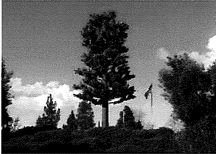
Image 3: Example of a pine tree cell tower design (Image retrieved from Cell Trees Inc.: http://www.celltreesinc.com/pine-trees.html )
