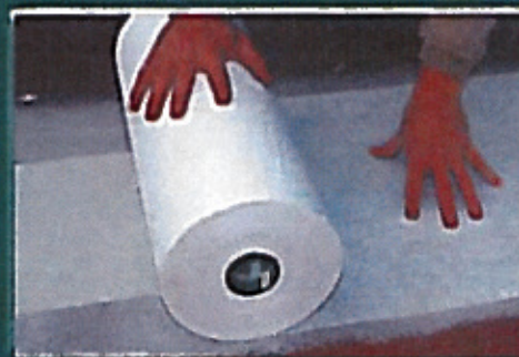
STEP 6: Install wide ARMOR® fabric
