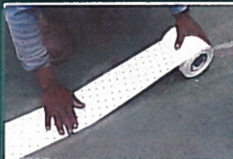
STEP 3: Apply ARMOR® release tape
