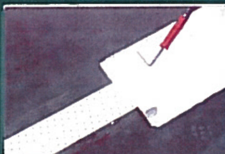
STEP 4: Apply liquid adhesive
