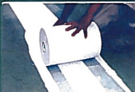
STEP 5: Install narrow ARMOR® fabric
