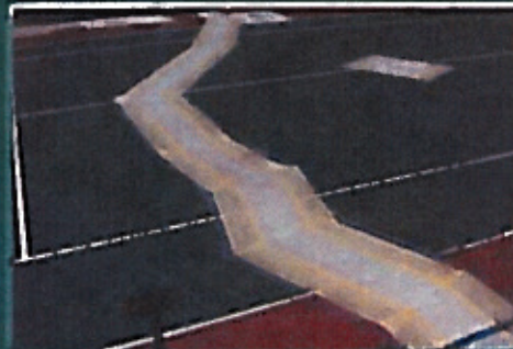
STEP 8: Finished...ready to color coat!
