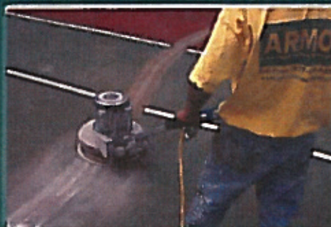
STEP 2: Sand flush to surface
