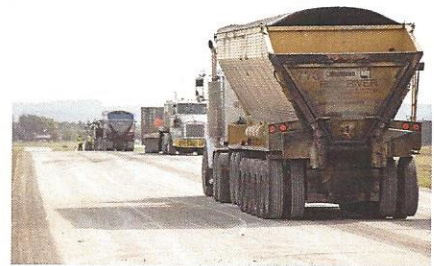
Taxiway A Rehabilitation
