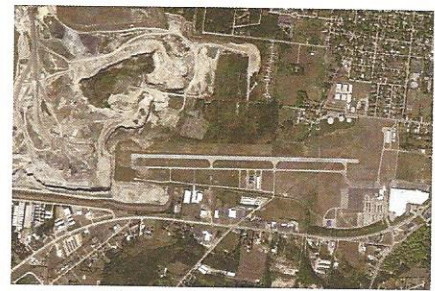
An existing quarry to the west of CVX adds challenges to future planning at the Airport.
