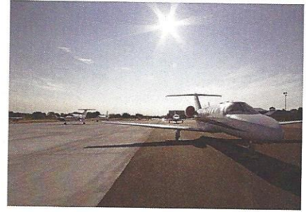
South Taxilane Construction
