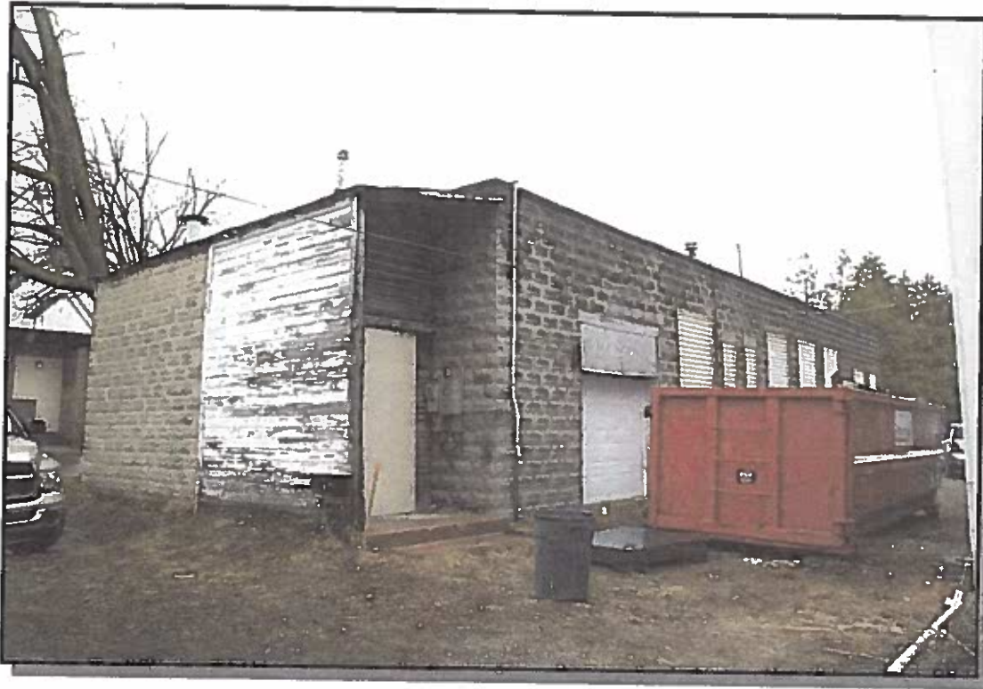
Rear Elevation Facing NW
