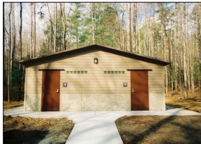
Men /Women ADA Restroom and Rear Showers
