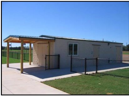
14' x 36' Restroom & Concession Facility
