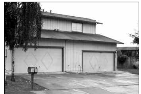
Above: UNDESIRABLE These residential projects are POOR design examples. Their parking, garage doors and driveways dominate the neighborhood.
