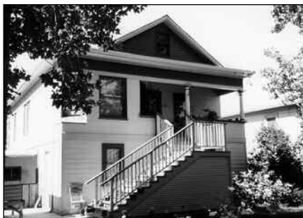
Above: UNDESIRABLE This cottage was raised a full level requiring the front stairs to “dog-leg” away from the sidewalk.
