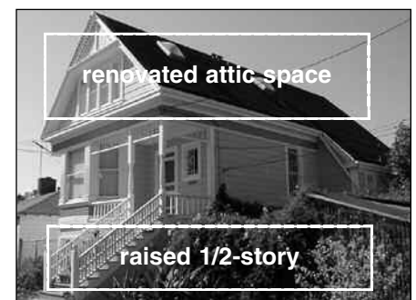
Above: DESIRABLE This cottage was raised 1/2-story to make room for a lower level floor. The project also included improving attic space.
