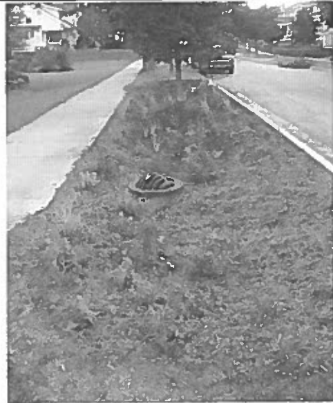
This is one of the recently completed rain gardens incorporated into the Park Avenue storm drainage system.
