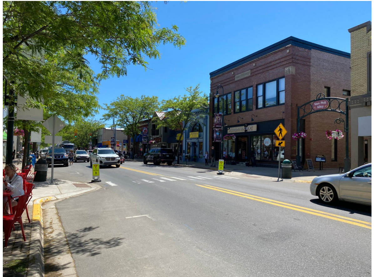
Mid Block crossing at Bridge St.
