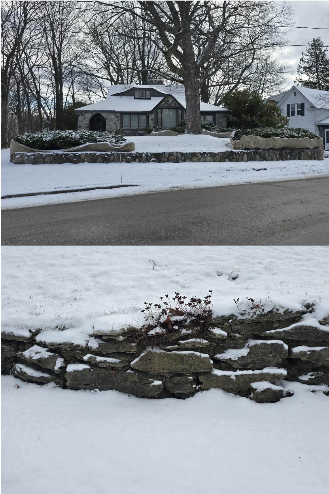
Existing stone wall 304 Park Ave
