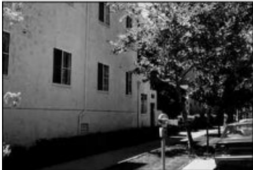
Above: UNDESIRABLE These apartment buildings have ground level parking and a tall blank wall along the street. The design is out of scale with the adjacent buildings. The architecture is spare and unattractive.
